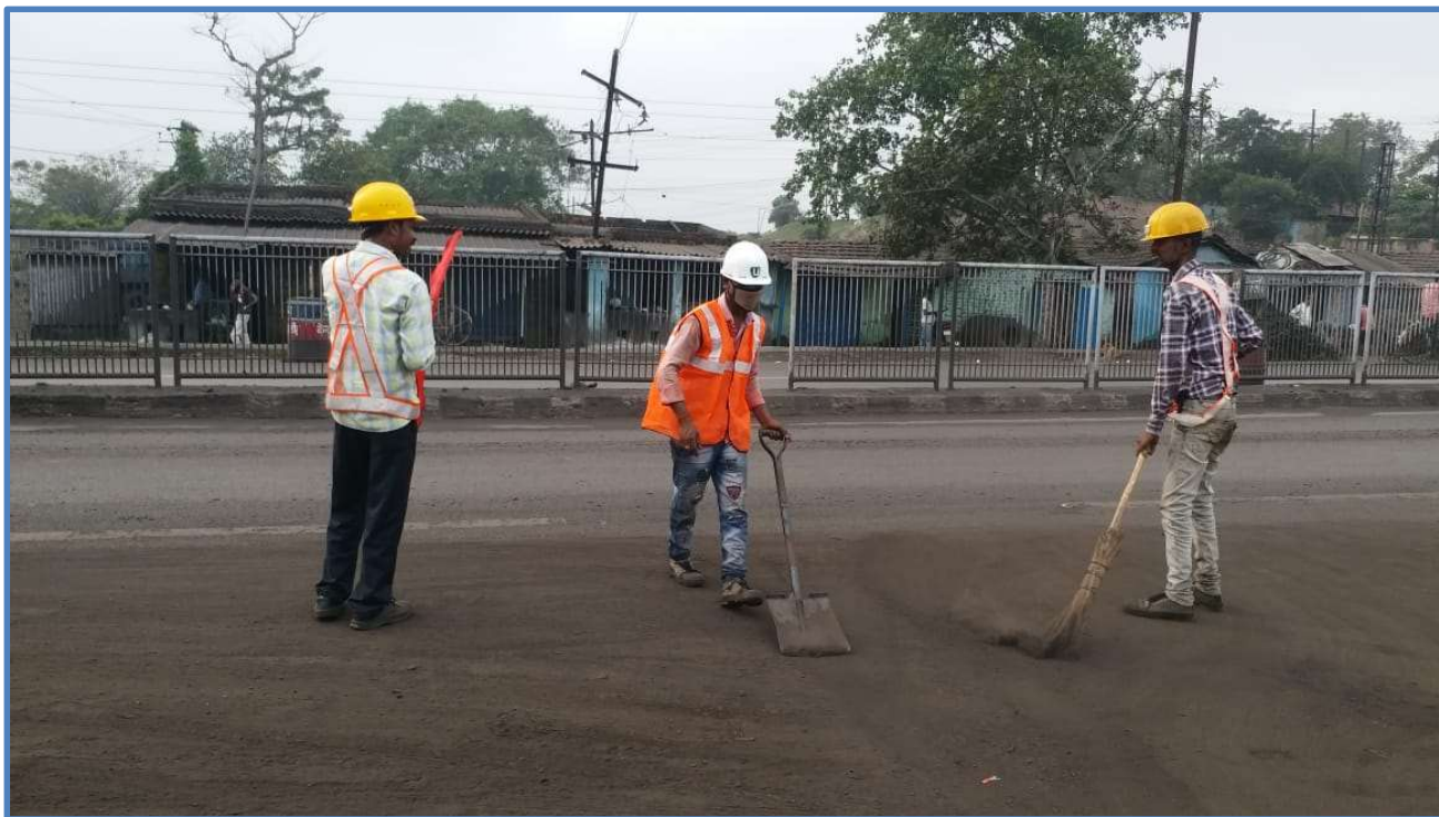
Picture 3 – Manual Sweeping of Public Road
